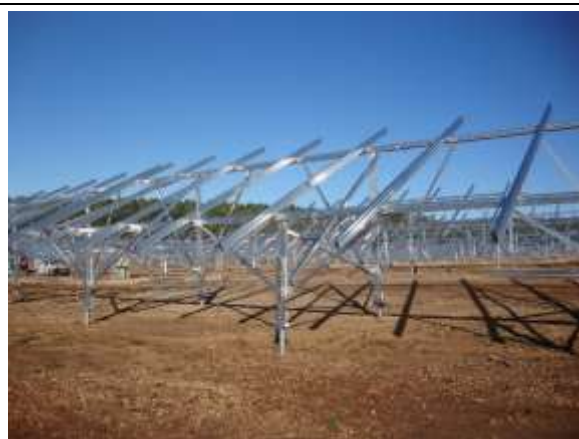
Photo 5-1 Typical anodized aluminium frame
