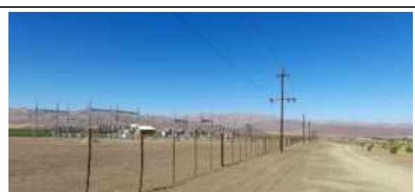
Photo 5-6 Existing power line to be upgraded
